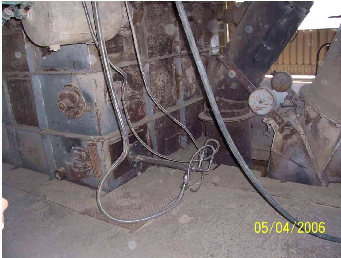
FIGURE 3 SNCR ammonia injections.
