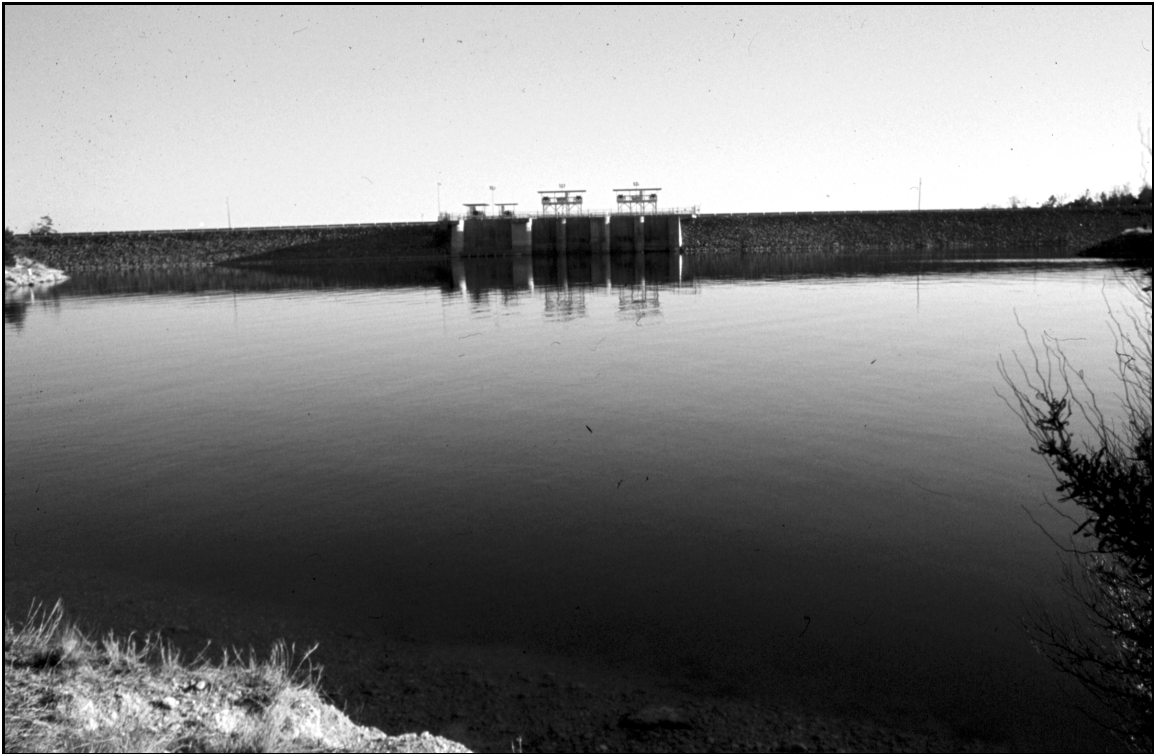
Spillway at Sam Rayburn Reservoir
