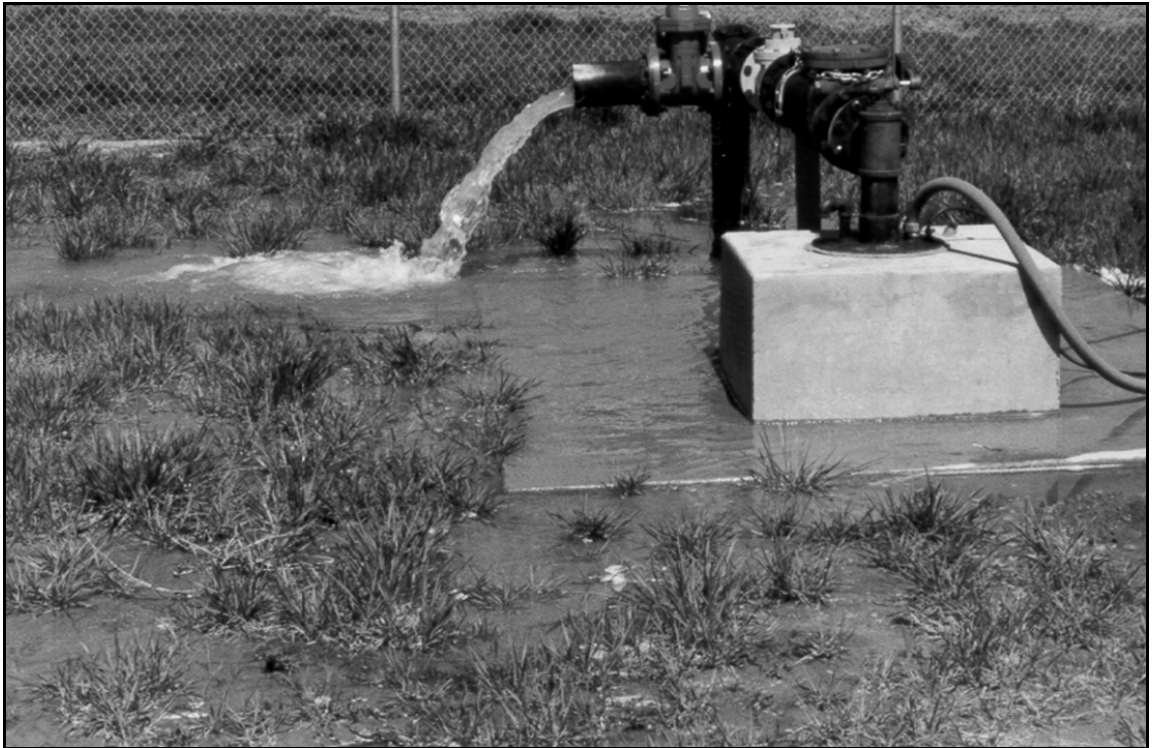
Groundwater well in City of Friona
