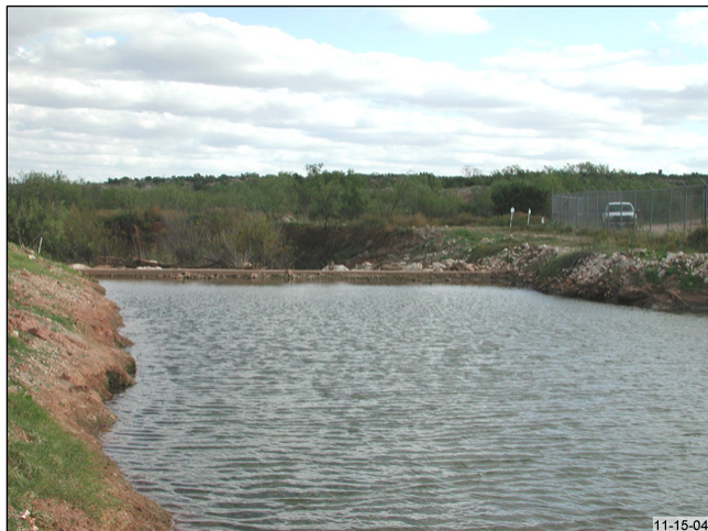
Figure 6: Beals Creek Pump Station southeast of Big Spring
