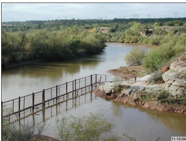
Figure 7: Colorado River Pump Station northwest of Colorado City
