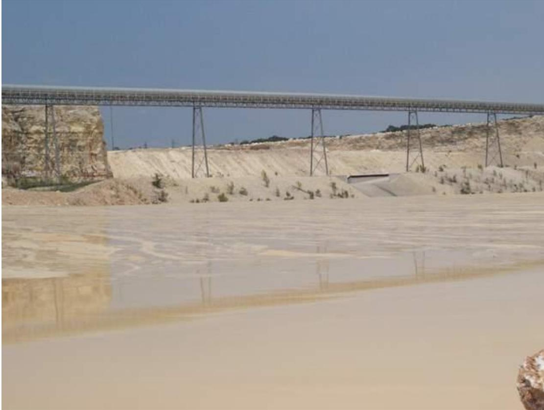
**Figure 2.** Large-scale sedimentation basin at aggregate quarry.
