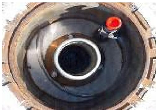
Figure 1. Spill bucket.
