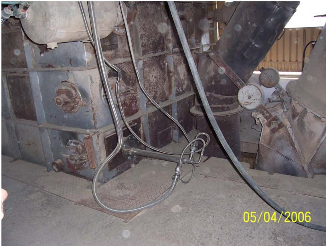
The most recent catalyst cleaning system utilizes preheated compressed air that continuously cleans the catalyst. Dry compressed air of about 900m<sup>3</sup>/ hr at 10 bar pressure passes through a heat exchanger coil that is located in the seventh stage of the SCR reactor, and then passes through insulated lines to each stage/layer of the reactor. Then the air passes into the reactor where a series of nozzles are located on two parallel bars, which span the width of the reactor.
