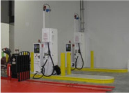
Sysco Corporation contracted with Air Products to supply hydrogen and hydrogen fueling technology for Sysco's new, 585,000 sq. ft. distribution center in Houston, Texas. The fueling station is used to fuel a combined fleet of over 100 hydrogen fueled pallet and reach trucks used in daily operations.
