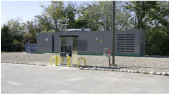
Hydrogen fueling station. University of Texas Pickle Research Center, Austin, TX. Reformer, processing, storage. System can produce 60 kg per day. 2009. To advance commercialization of hydrogen-powered transit buses and supporting infrastructure.
