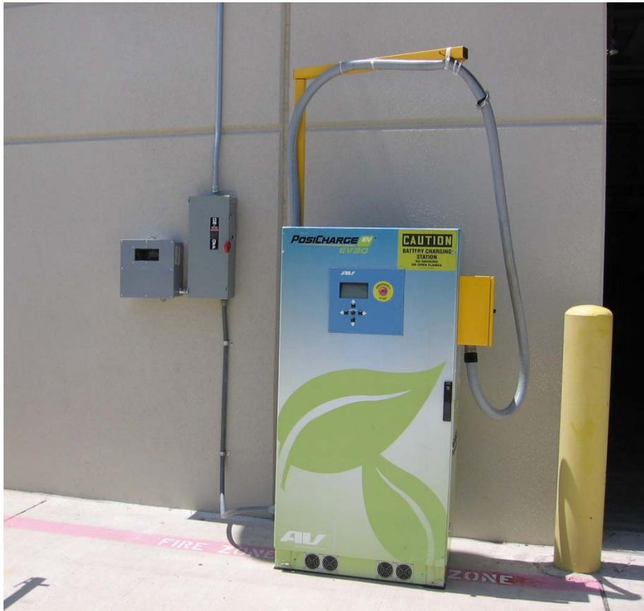
Operational checkout of the charger was completed on May 28, 2012, after Proterra completed software upgrades that were necessary to recharge the batteries on the bus. The batteries were connected to the charger at 44% state-of-charge (SOC) and were recharged overnight to 95% SOC. The electrical energy consumption during this charging event was 28 kilowatt-hours.
