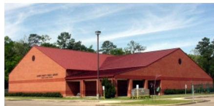
North Channel Branch Library
