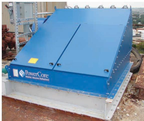
CPV-12 - Cement silo bin vent conveyor 3,700 cfm (6,285 m³/h)
