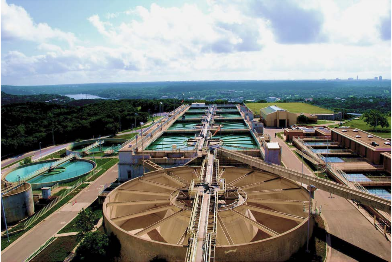
Albert H. Ullrich Water Treatment Plant, Austin, Texas
