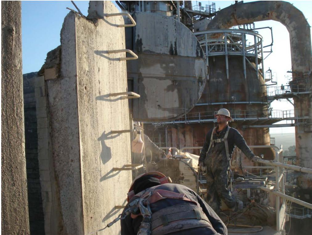
Photograph 2 – Workers Remove Stack Wall with Saw
