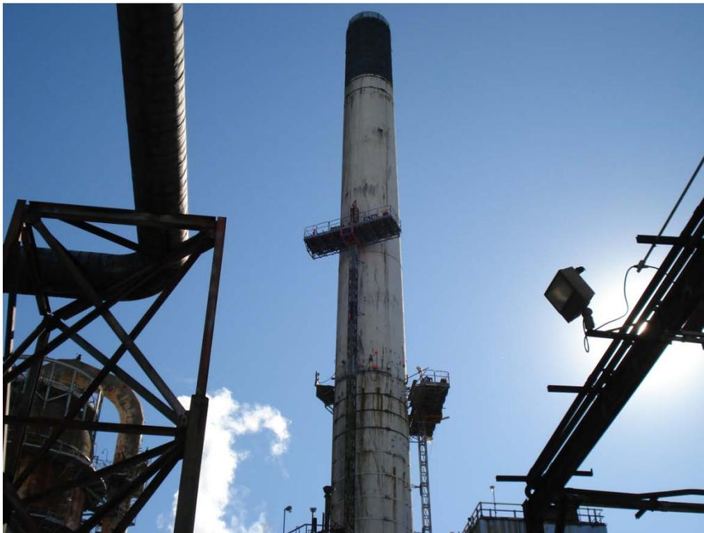
Photograph 1 – Mast Climber Scaffolding Being Erected
