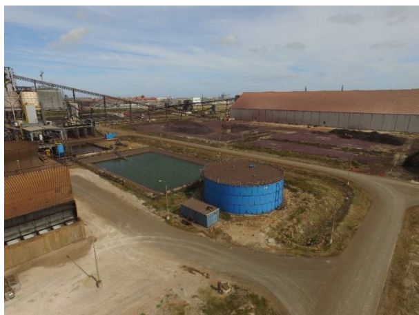
Figure 6.1.2: Before Phase 1 Construction
