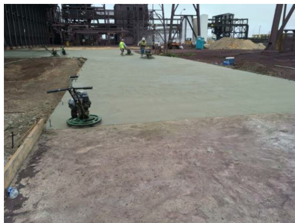
Figure 6.1.3: Phase 1 in Construction
