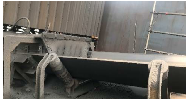
Figure 4.3.4.2 – TT24 Lower Transfer Point
