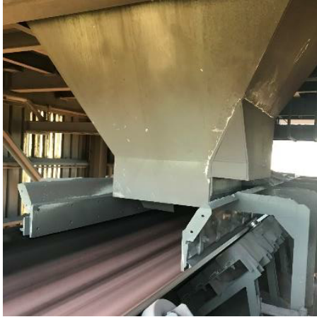
Figure 4.4.4.1 – TT23 Lower Transfer Point
