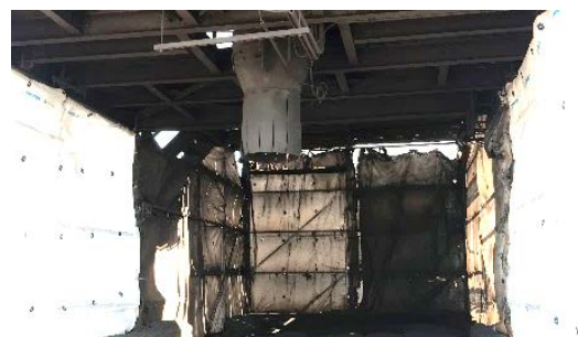
Figure 4.4.2.1 – TT22 Lower Transfer Point
