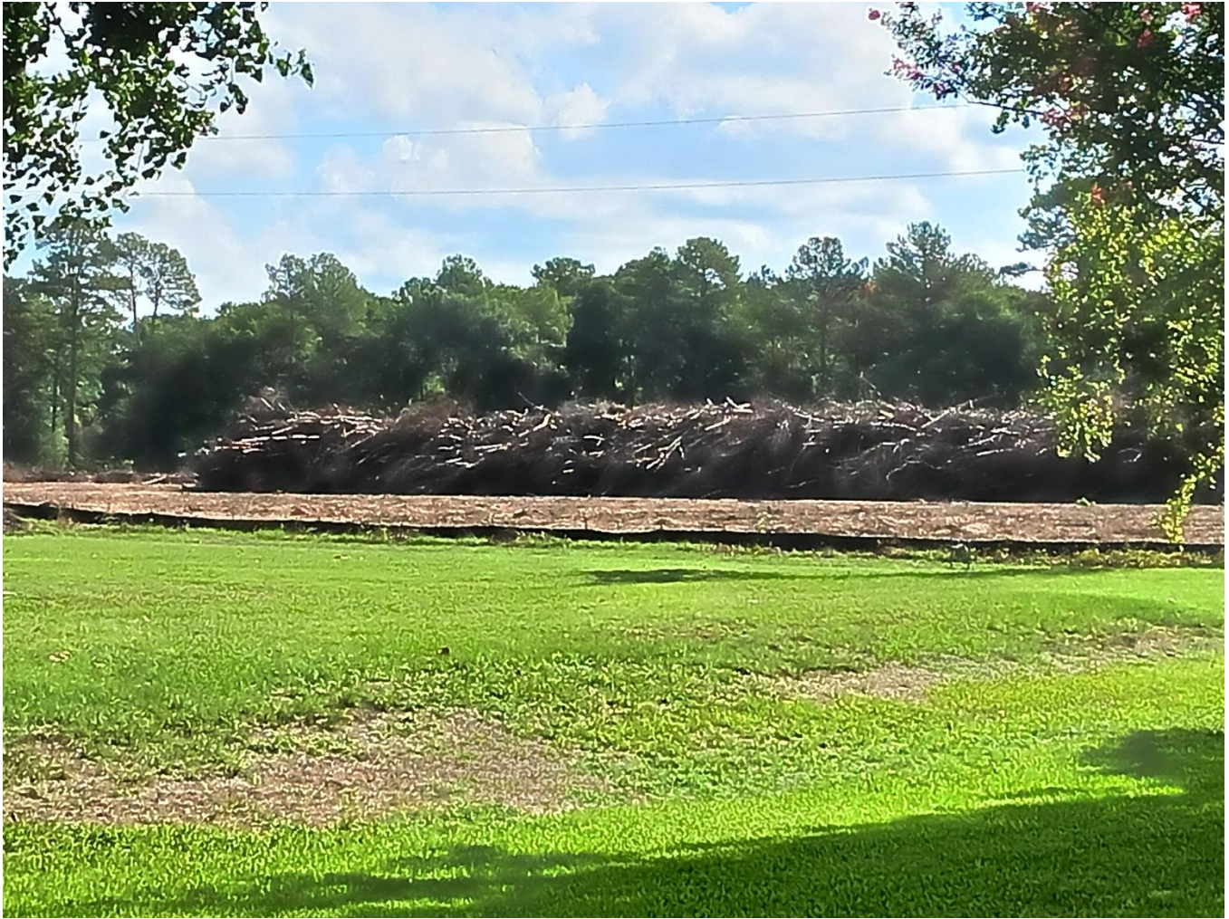
Current view of development progress (facing east from 22603 Three Pines Drive)
