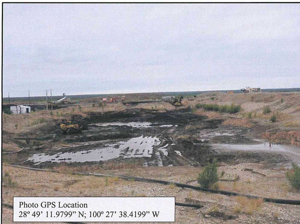
Photo 4. Pond RP-2 clean-out/maintenance operations by new landowner (view to southeast).
