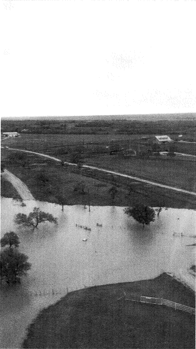
Pictured Above: Flooding on Morrison Creek covering SE River Road in Martindale. October 2015
