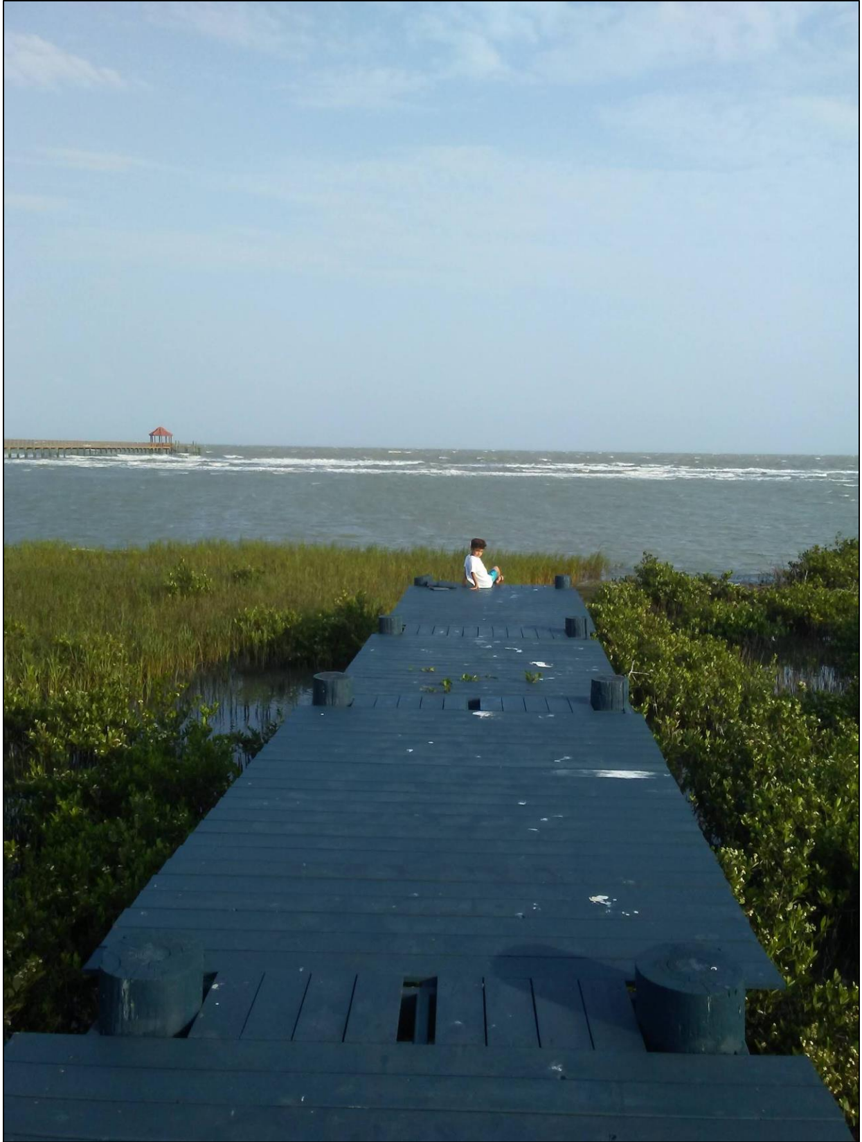
Photo 4: End of the pier extending from Mr. Encarnacion Serna's property into the Corpus Christi Bay.
