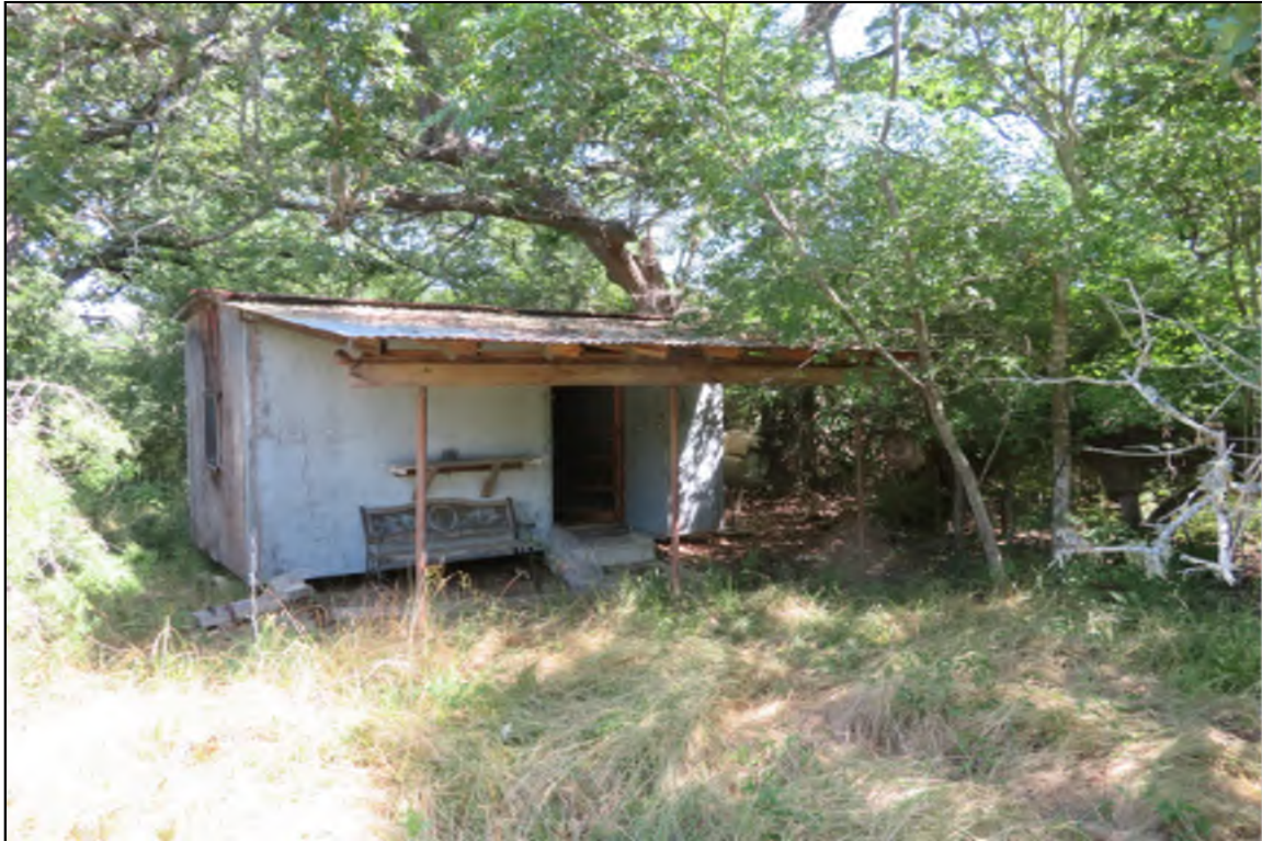
Photo 8_ View of the cabin located on the property looking north.
