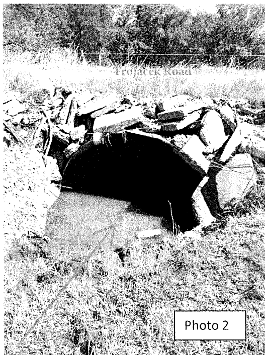
Photo 2: existing culvert pipe for Four-Mile Creek crossing Trojacek Road
