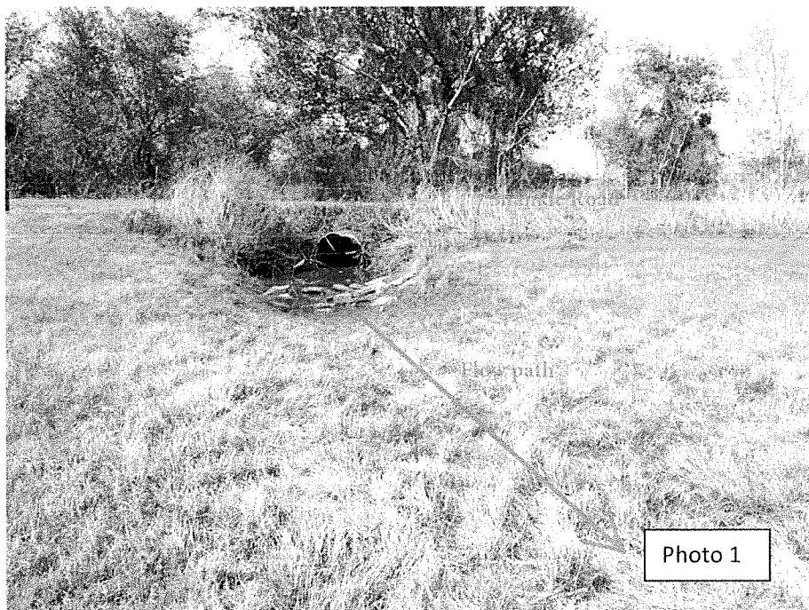
Photo 2: existing culvert pipe for Four-Mile Creek crossing Trojacek Road
