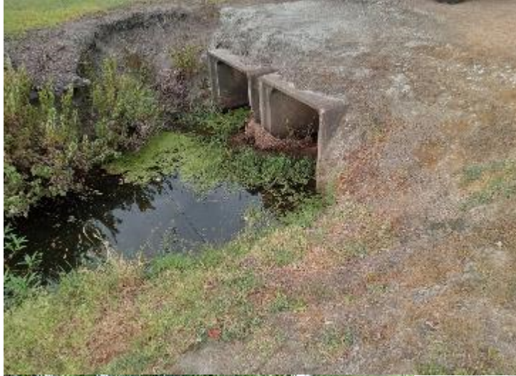
Photo 5C Closeup of 2 x 36 inch box culverts under Madeline St. to the West
