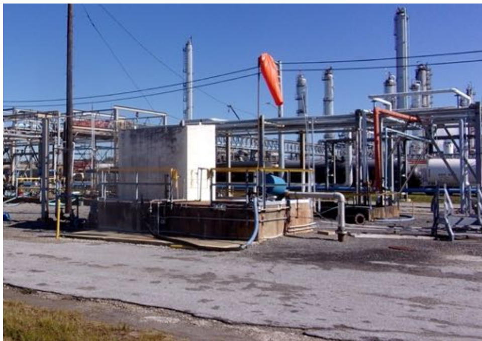
19. Outfall 101 septic chlorinator
