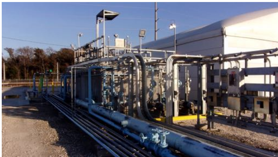
20. Outfall 201 septic chlorinator
