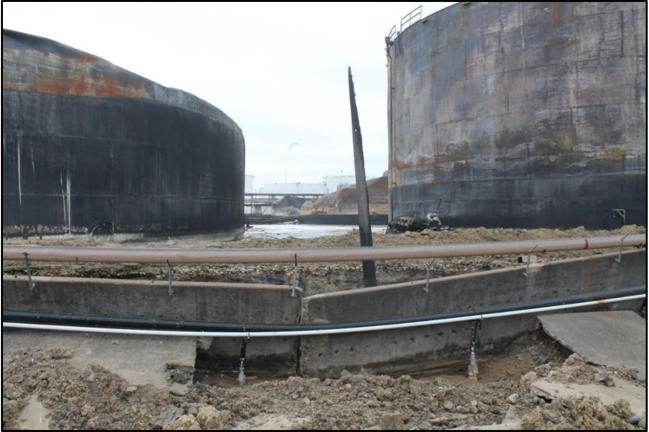
Figure 17. Close-up view of the First & Second 80's tank farm containment wall breach that occurred on Friday, March 22, 2019. (Credit: HCFMO).
