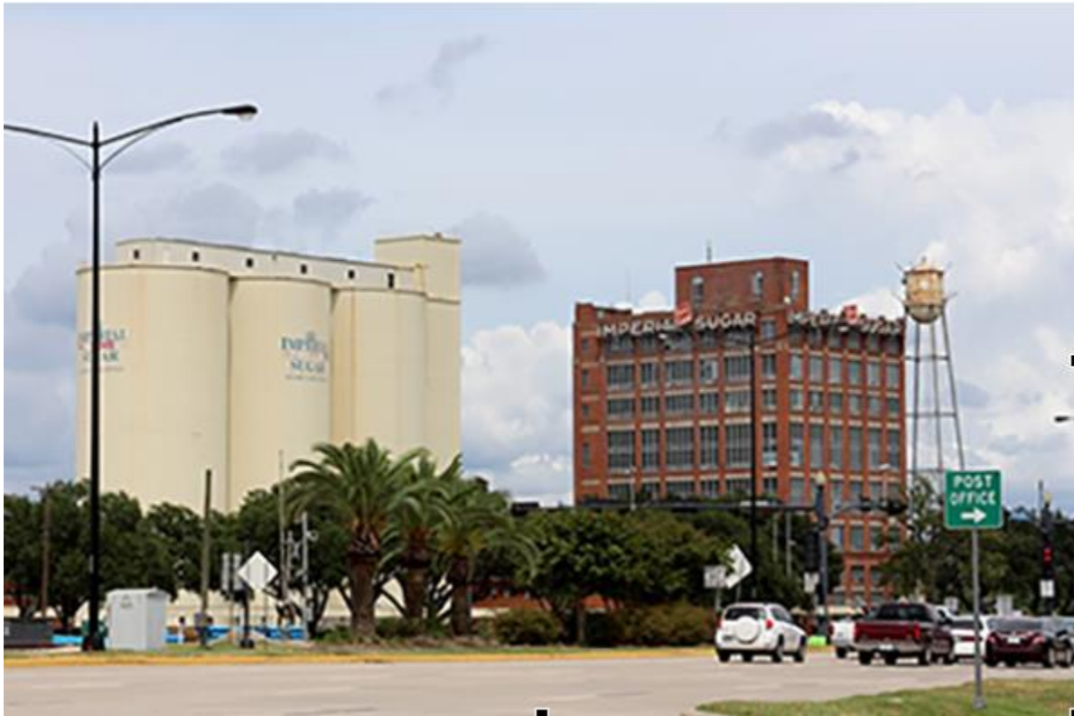
Figure 1. The former Imperial sugar refinery building and tanks.
