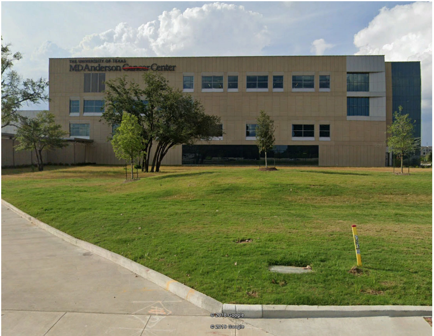
Site during construction in 2017; future site for MD Anderson Cancer Center
