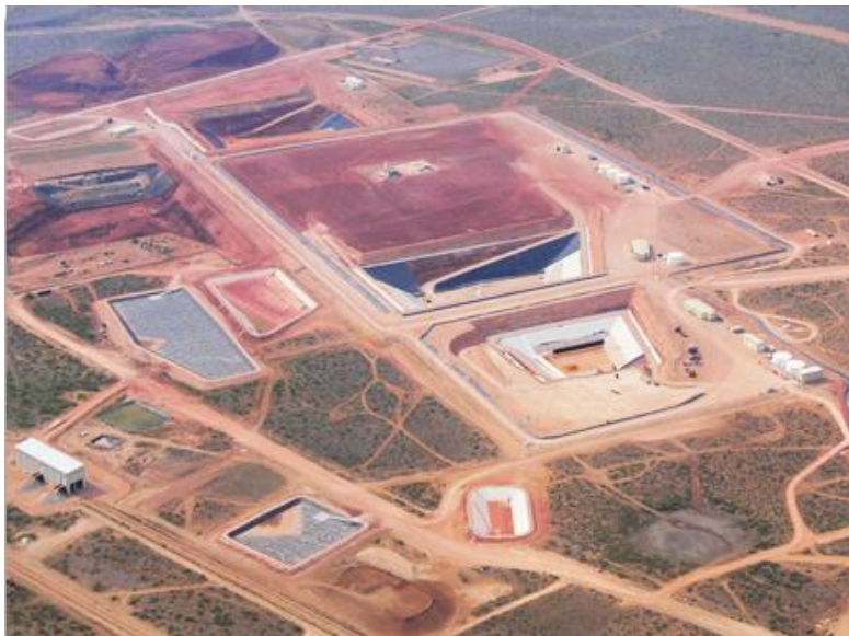
Figure 1. Aerial view of a Low-level Radioactive Waste Facility
