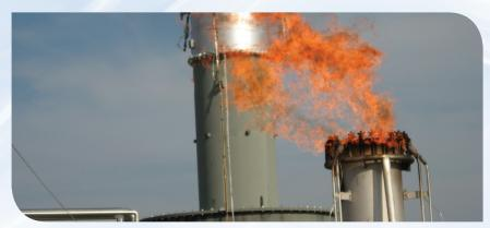
This is an example of a steam-assisted flare effectively burning and destroying waste gas (achieving high efficiency). Notice the flame.
