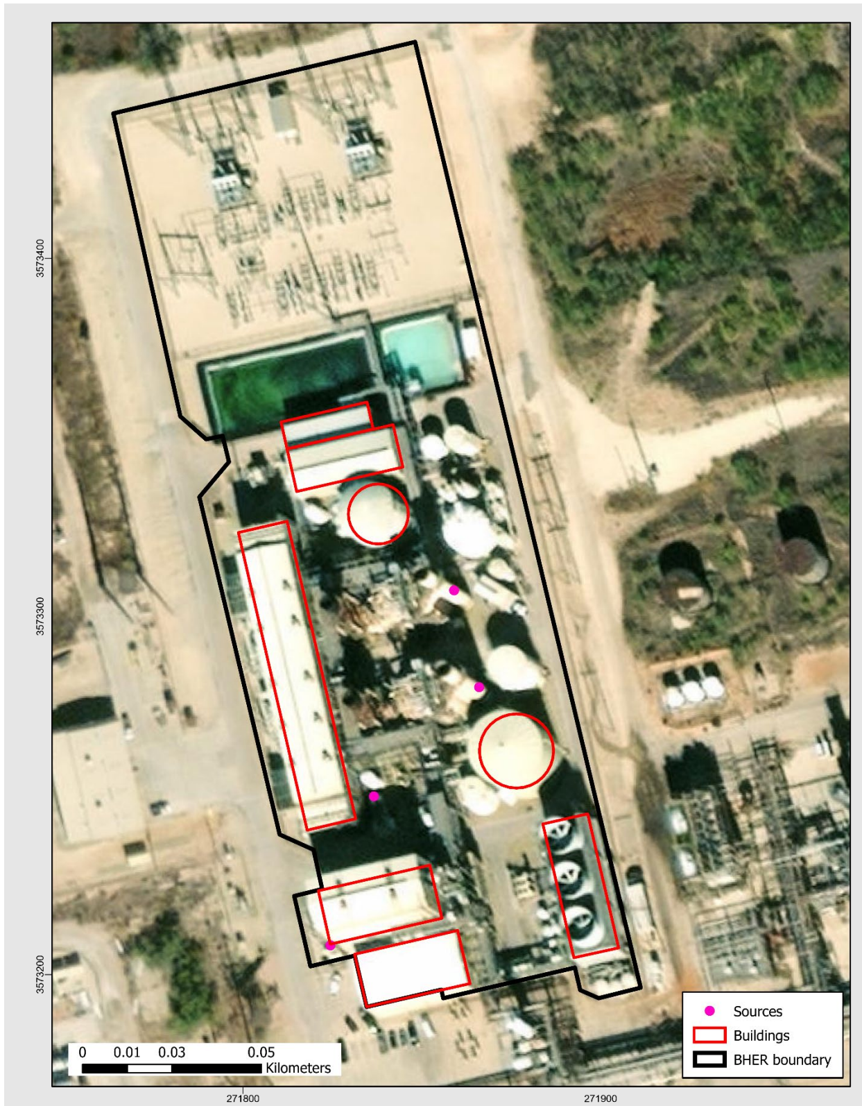
Figure 4-4: BHER C R Wing Cogeneration Plant Site Overview
