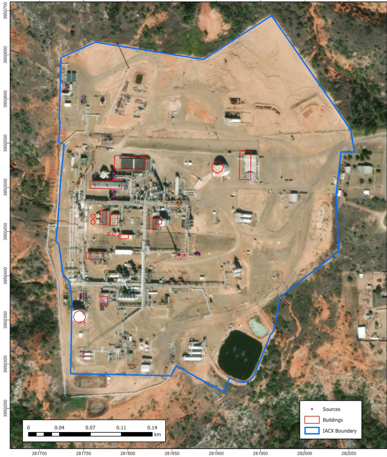
Figure 4-4: IACX Rock Creek Gas Plant Overview
