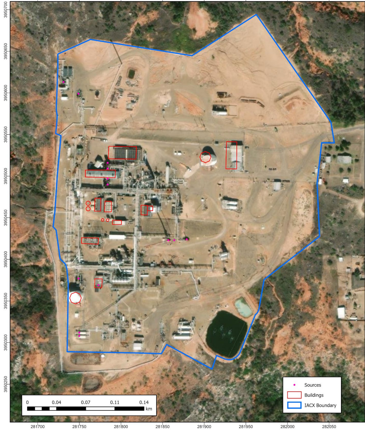
Figure 4-4: IACX Rock Creek Gas Plant Overview
