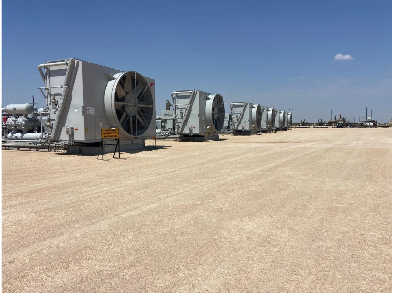
Figure 6- Completed Installation of Electric Compression
