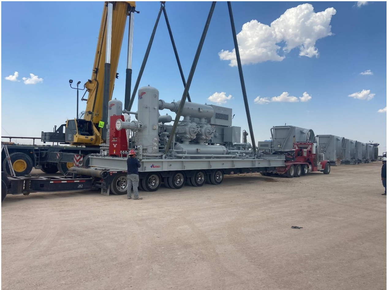
Figure 2- Unloading Electric Compressors
