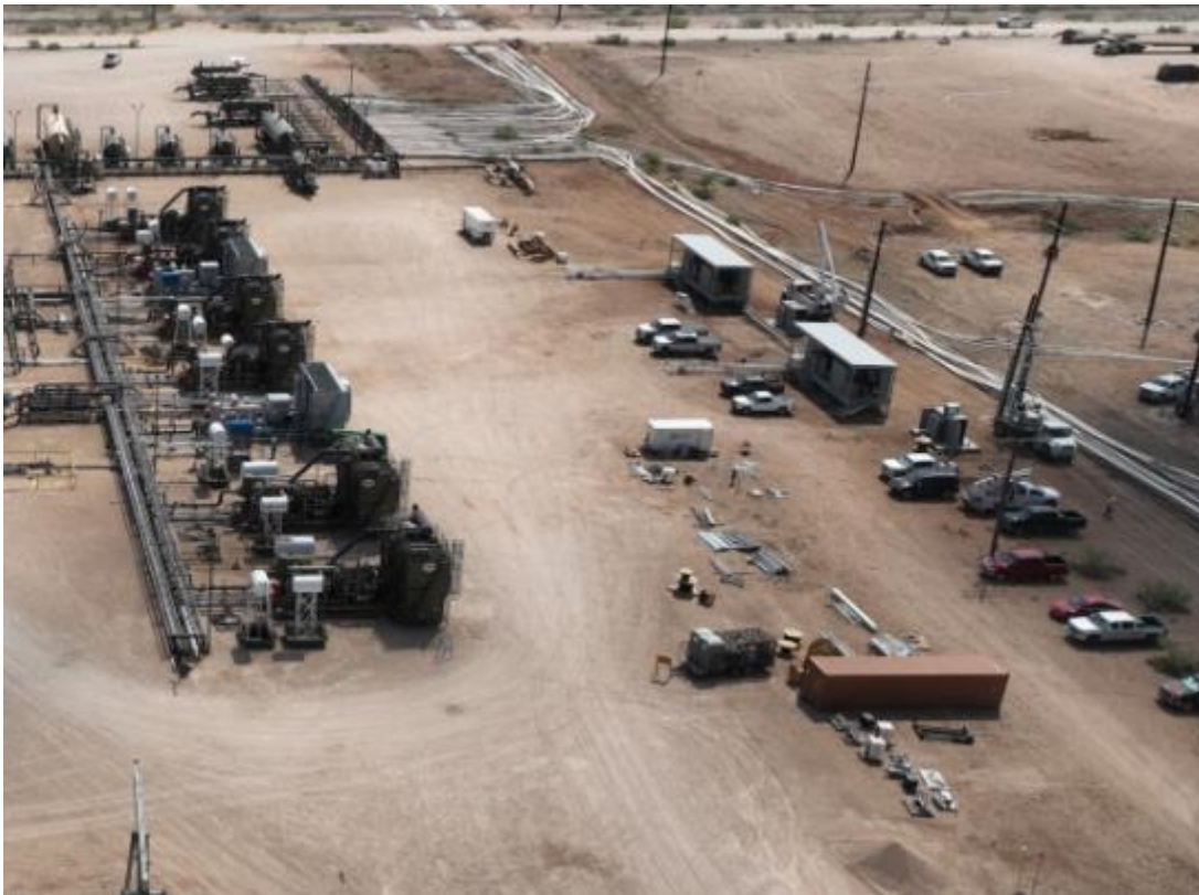
Figure 1 - Photo of Installed electrical equipment and powerline construction - May 12,2023
