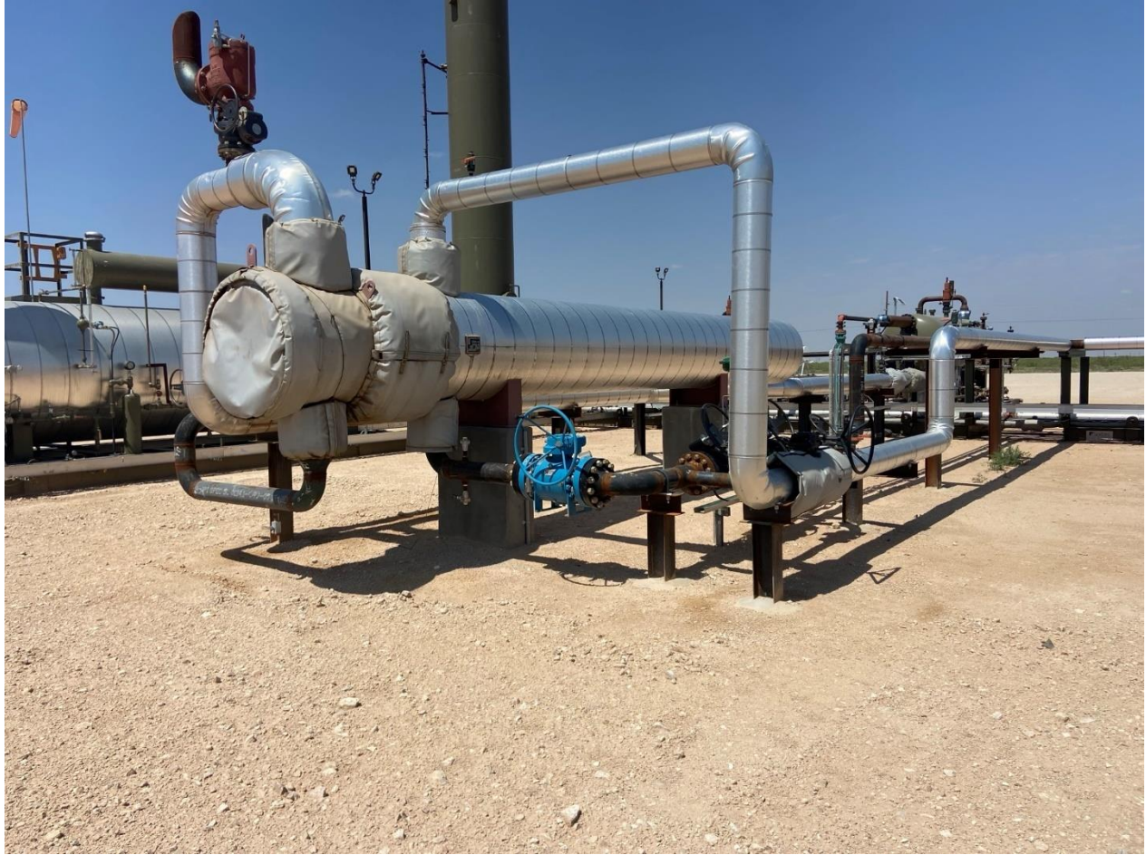
Figure 4- Heat Exchanger installation completed
