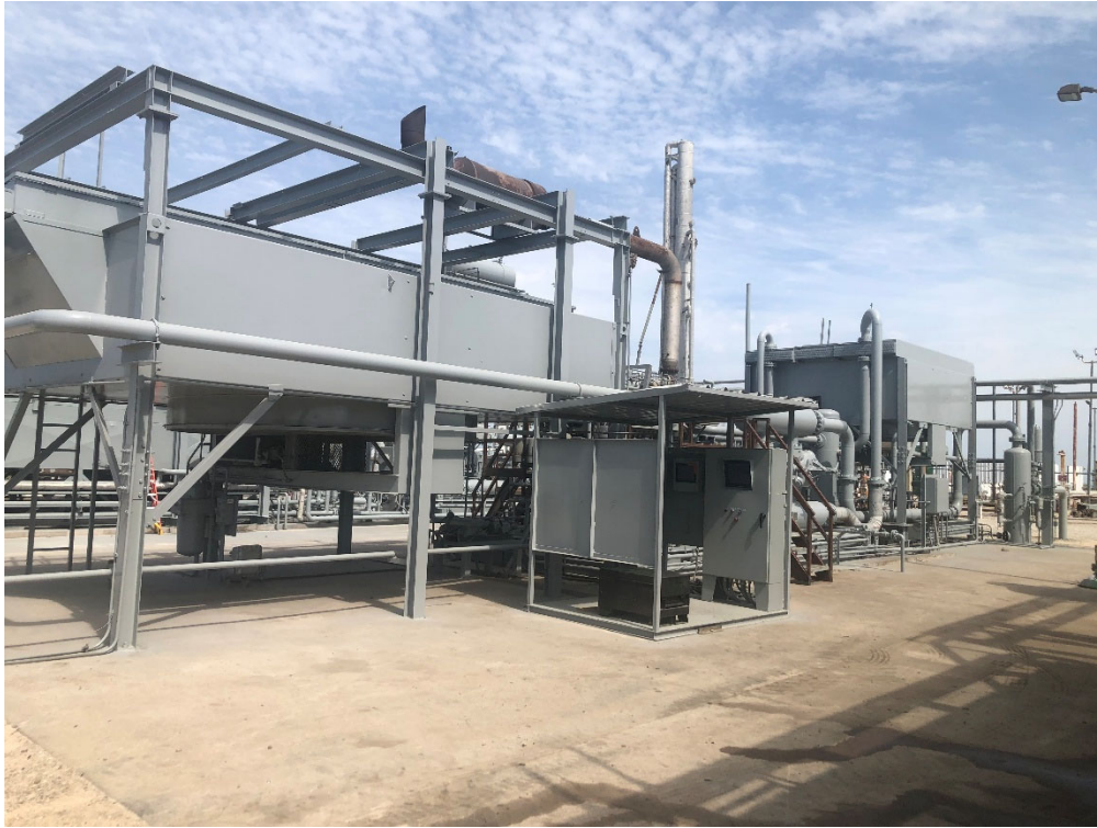
Completed # 3 engine with new engine control and PLC shown in the foreground
