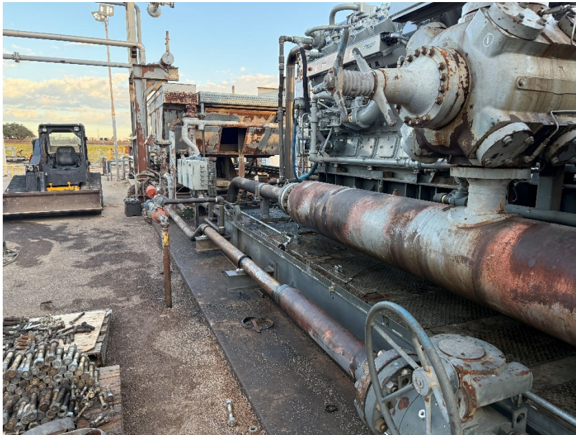
Refurbished compressor skid #3 installed in its slot
