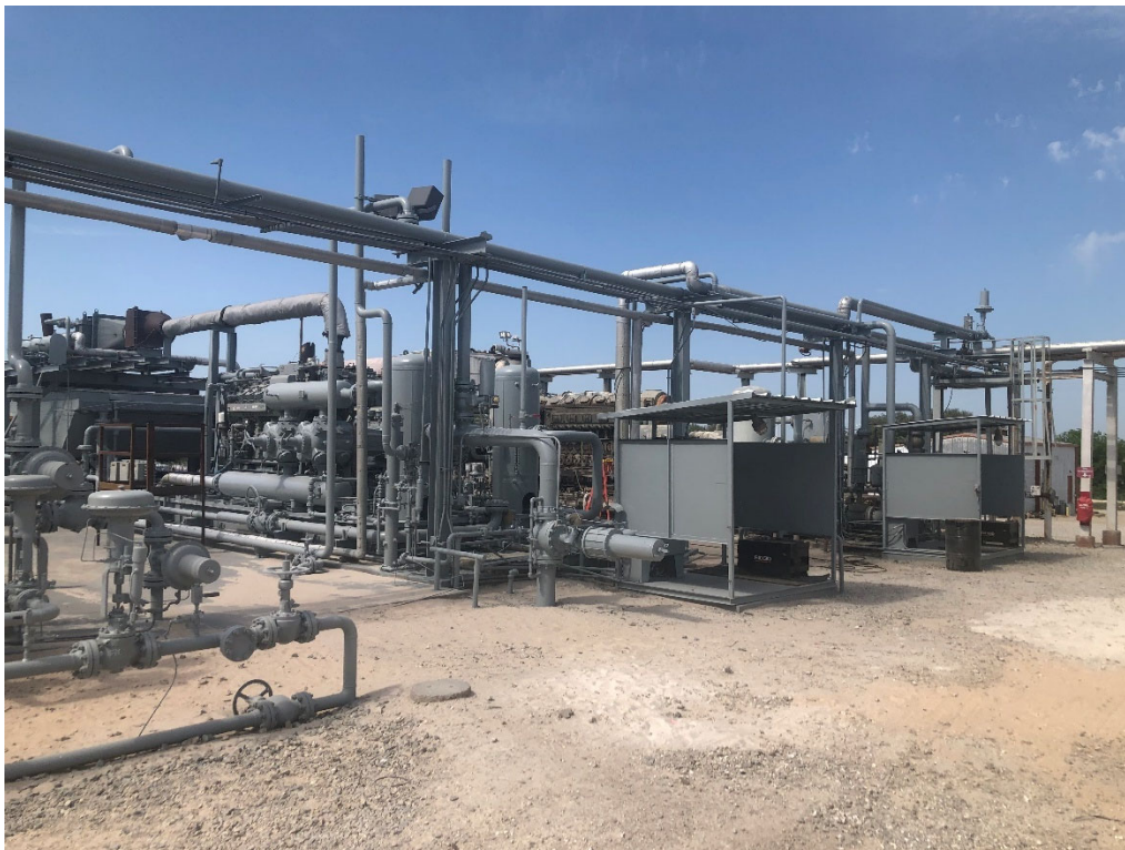
Completed # 2 engine - regenerative heater shown behind the catalyst housing
