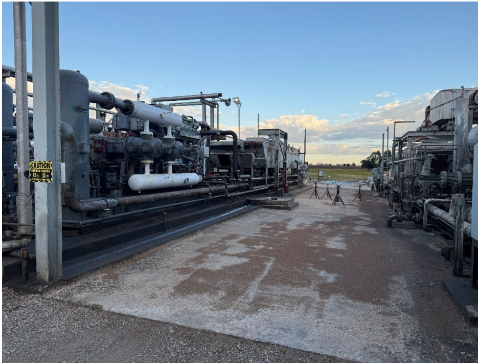
Both new engines set on the refurbished skids
