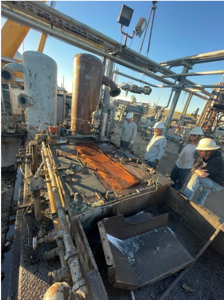
One of the old compressor skids after removal of the engine and compressor (compressor shown lifted by the crane in the background), prior to removal of the compressor skid
