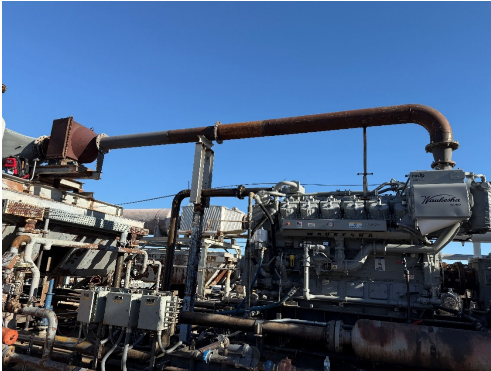
# 2 engine and exhaust – 3-way catalyst housing shown in the upper left, followed by the regenerative heater (grey)
