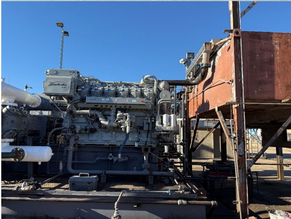
One of the new Waukesha 7044 S5 engines installed on the skid
