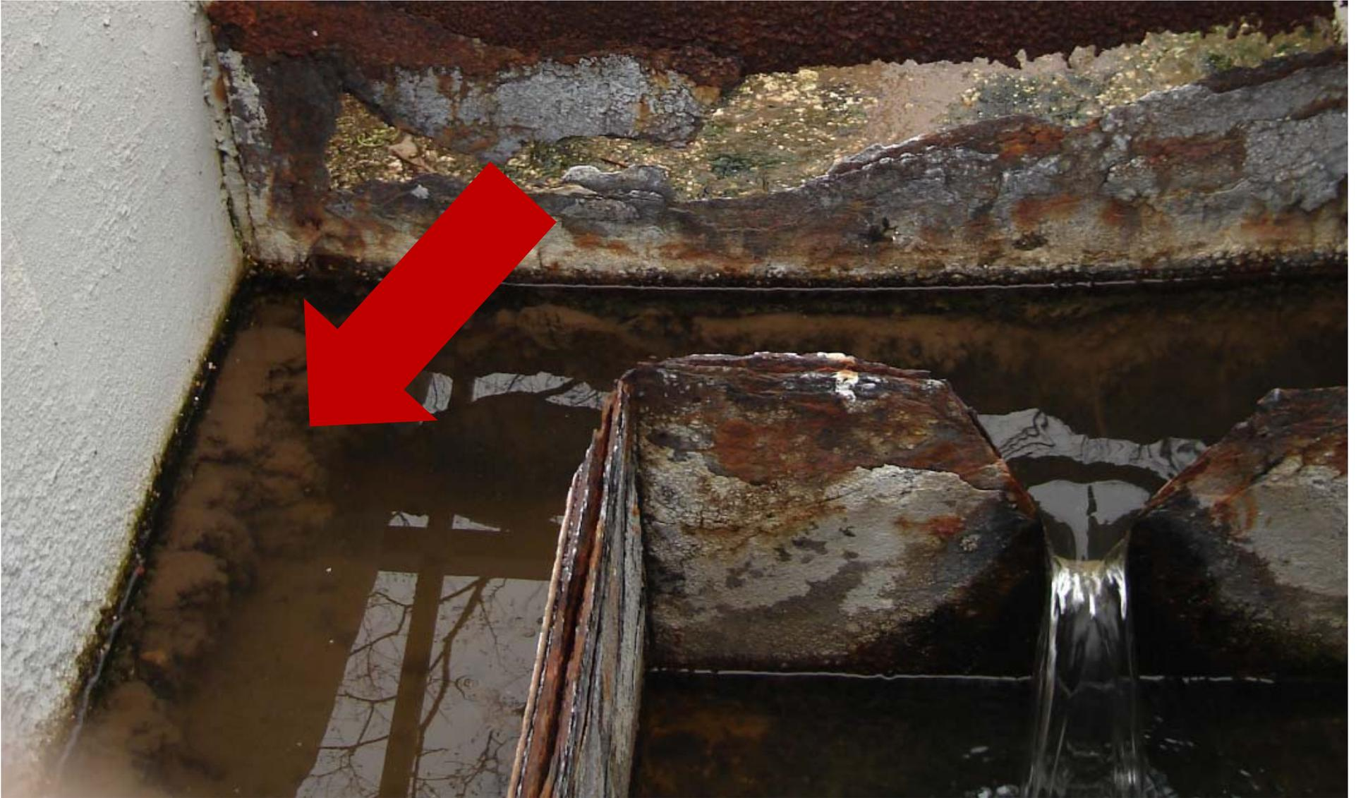
**Sludge settled in the chlorine contact chamber.
