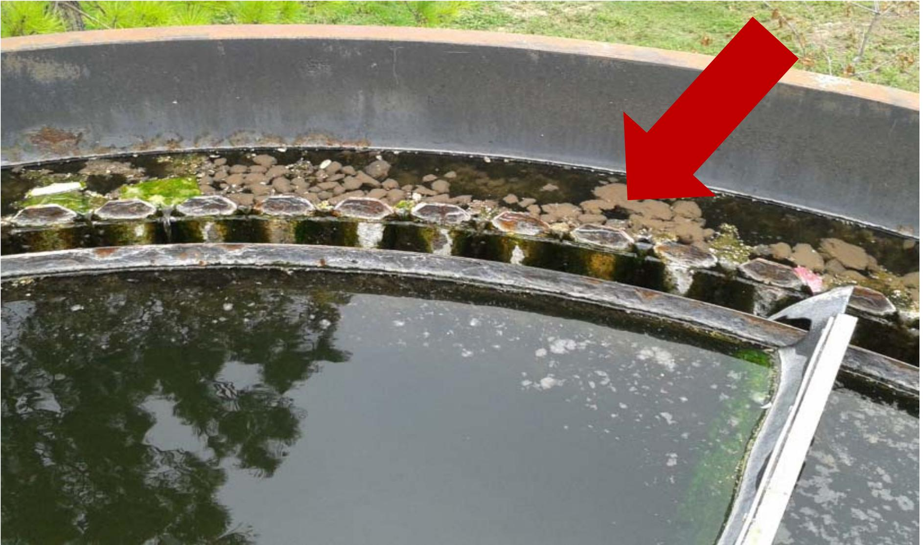
**Sludge rising in the clarifier. Increased suspended solids interfere with the disinfection process and increase bacteria counts in the effluent.**
