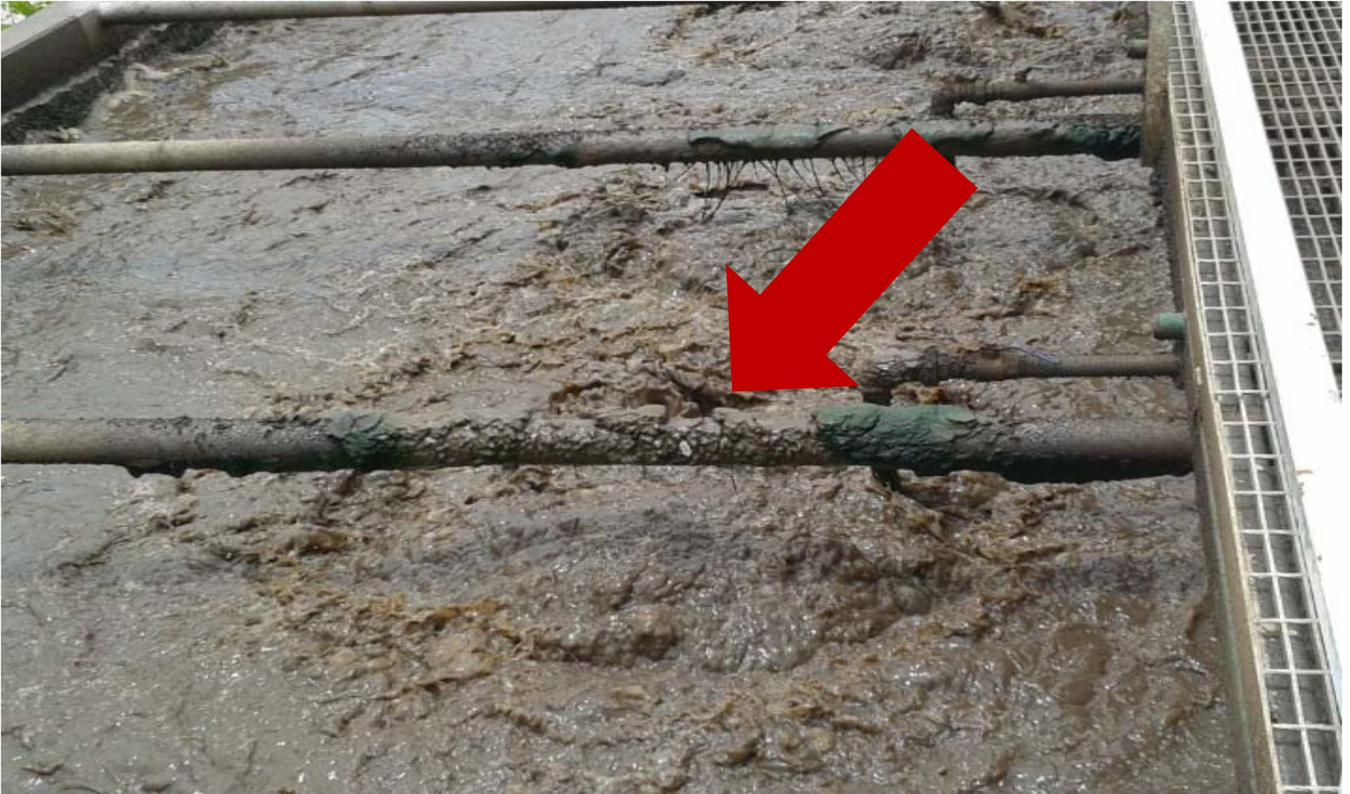
**Broken diffusers reduce dissolved oxygen levels in the aeration basin causing the microorganisms to become unhealthy or even die.**
