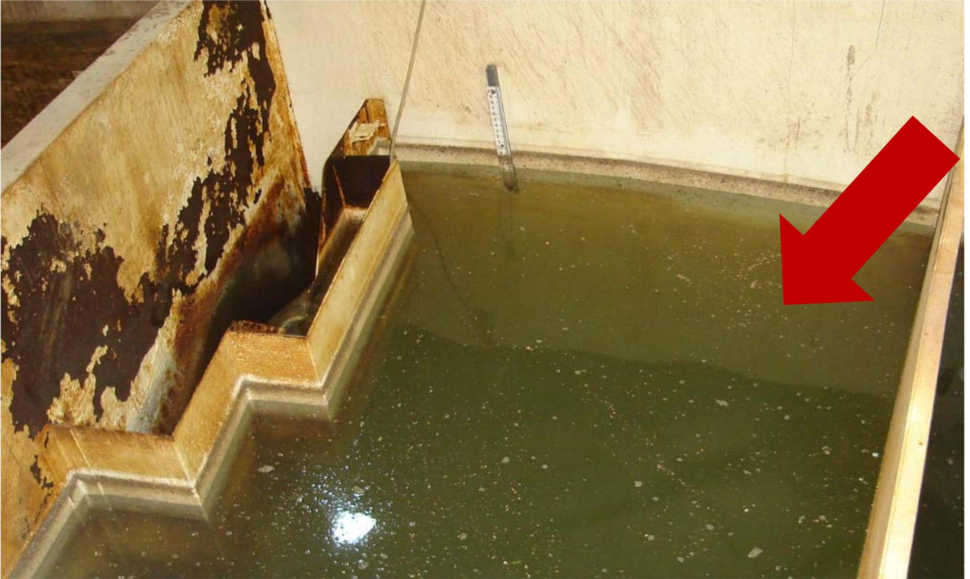
**Grease in the chlorine contact chamber.
