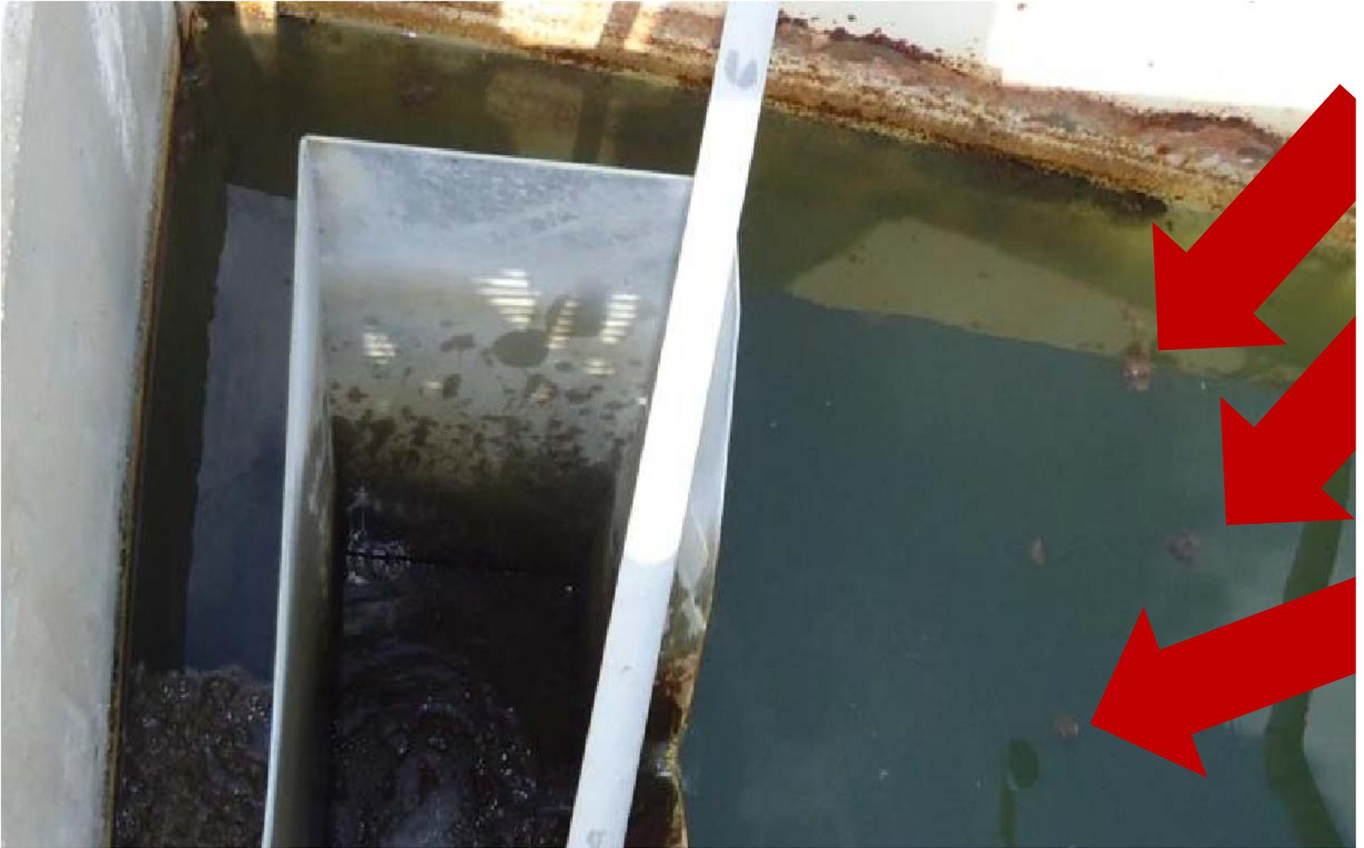
**Sludge clumps and grease reduce disinfection.**
