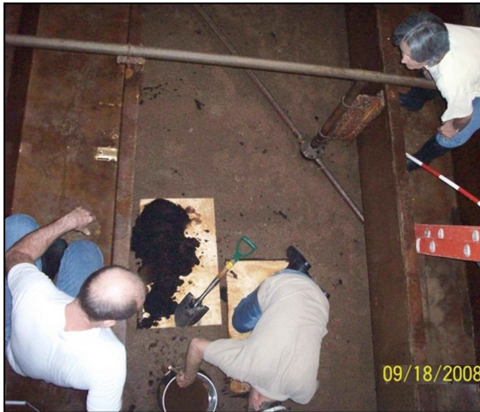
Figure 61: Checking for Media Stratification and Mudballs
