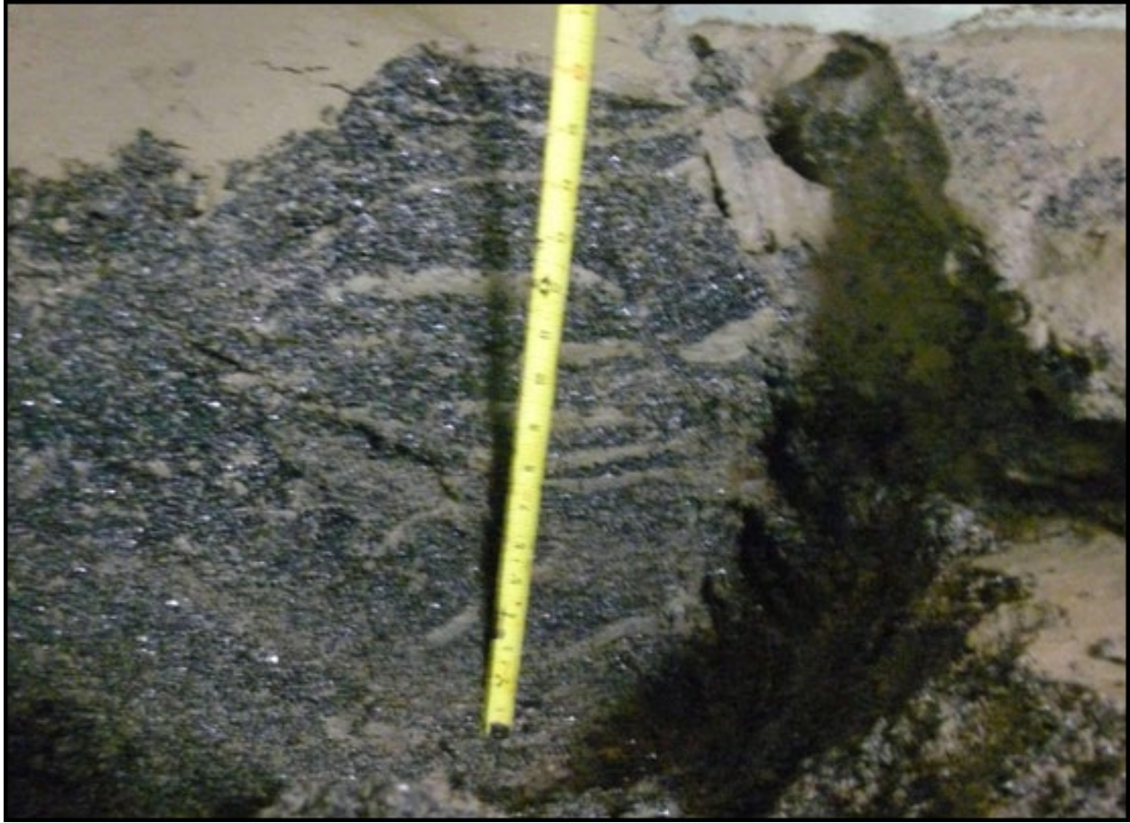
Figure 62: Mud in the Media Bed
