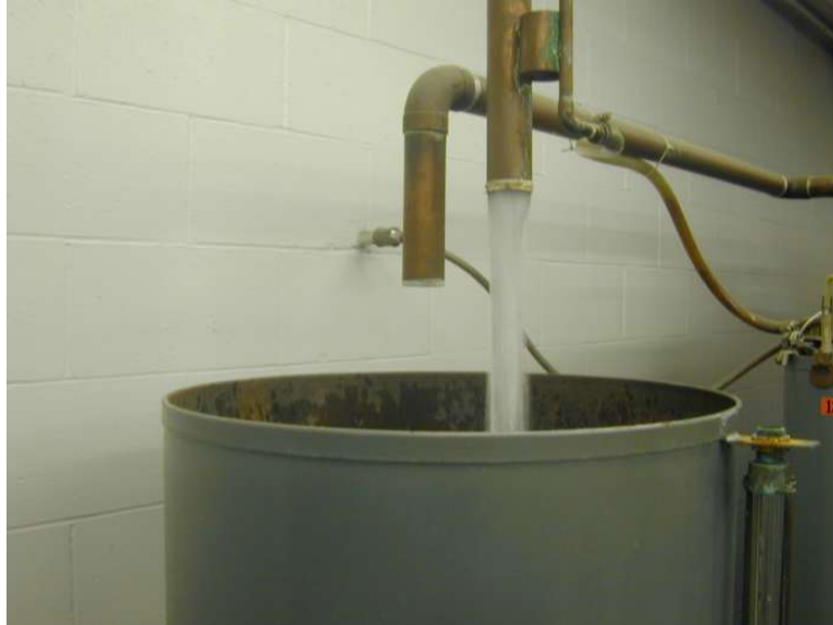
Figure 9: Photograph of air gap (AG).
