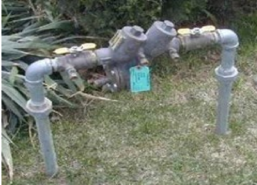
Figure 29: Photograph of a small RPBA
