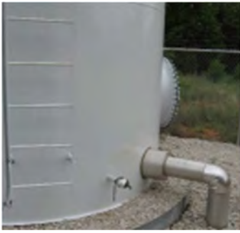
Tap on a ground storage tank (GST)
