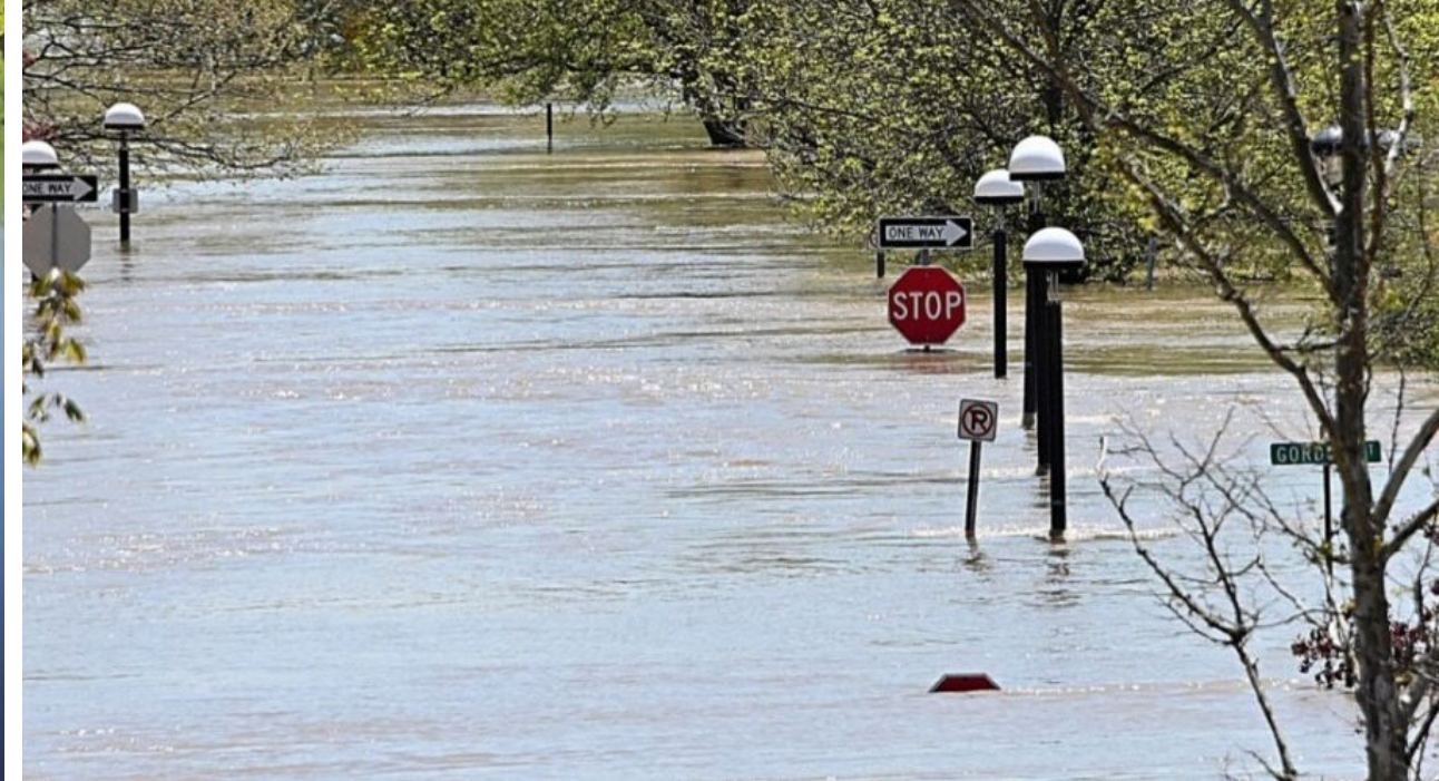
Central Michigan Dam Failures
