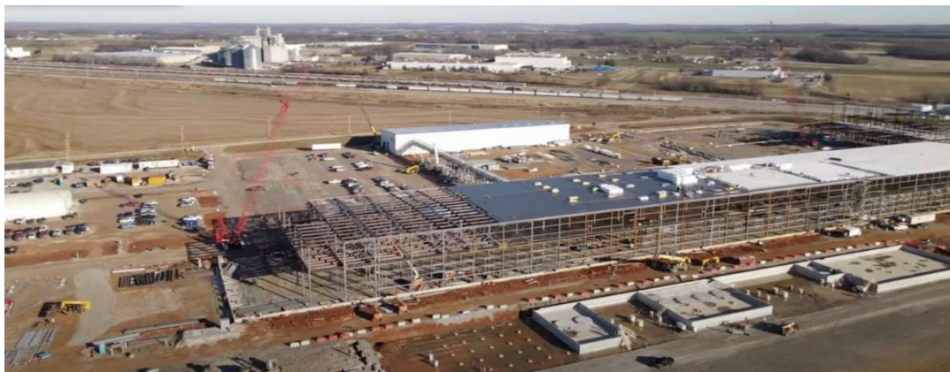
Ascend Elements' building under construction in Kentucky.
