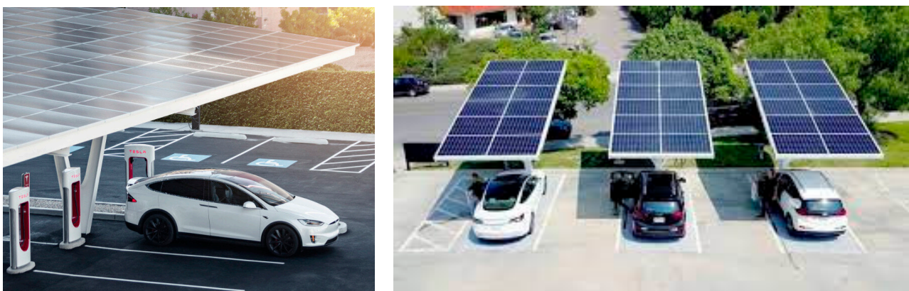
Figure 33. Off-grid solar-powered EV charger [71,72].
