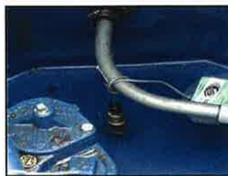
Liquid sump sensor
