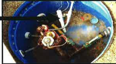
Sump sensor in contained turbine sump
