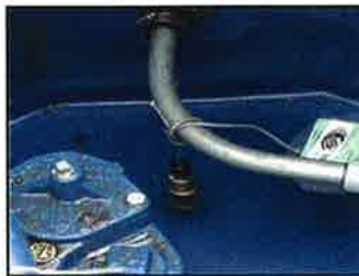
Liquid sump sensor
