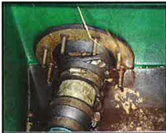
Sump penetration seals in poor condition
