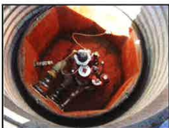
Dry, debris-free contained turbine sump
