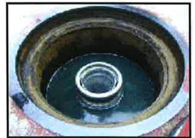
Spill bucket that contains liquid
