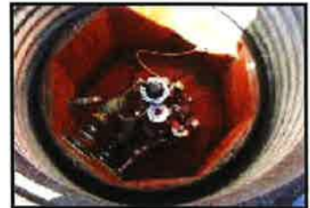
Contained turbine sump
