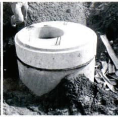
A "Prefab Manhole" Sealed In Four Minutes - Ready For Immediate Backfill
