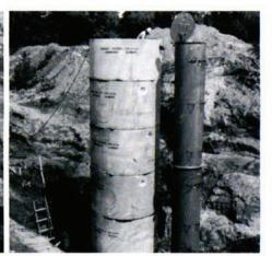
Typical RAM-NEK® Jointing Method For a 96" Concrete Pipe Wet Well, 42' Deep
