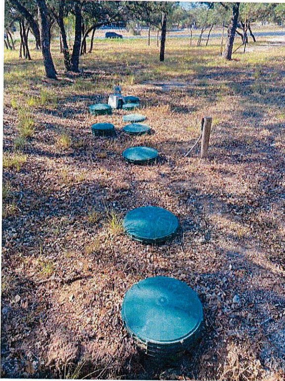
Photograph 1: Northwest facing view of the septic system feature MB-1.
