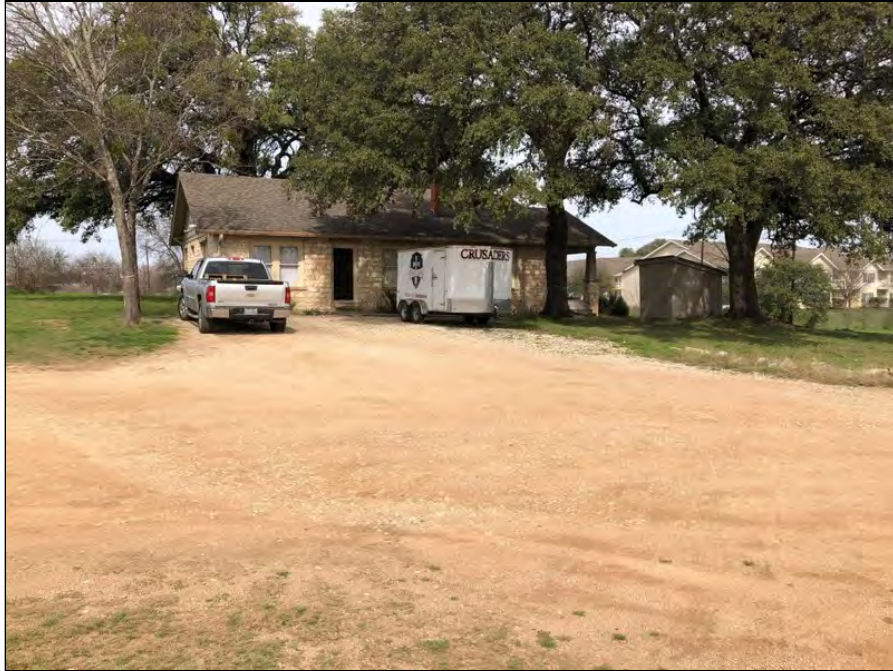
7 - View of permanent building and well pump house
