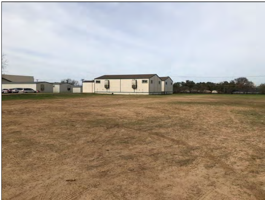
2 - View of western portion of subject property near temporary buildings
