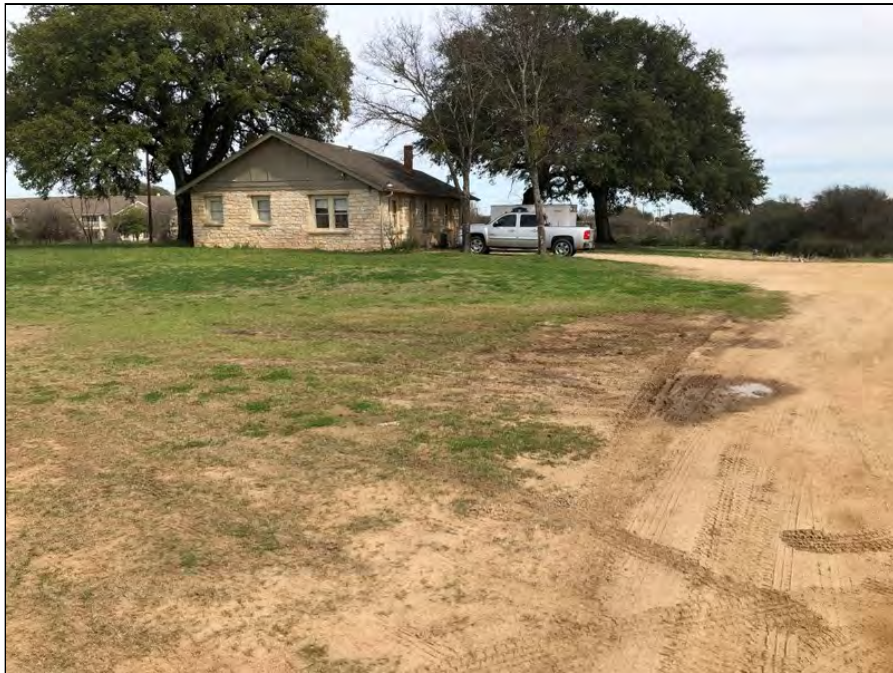
6 - View of permanent building
