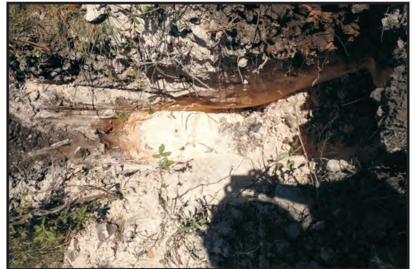
PHOTO 4 Close up view of F-2, after excavation
