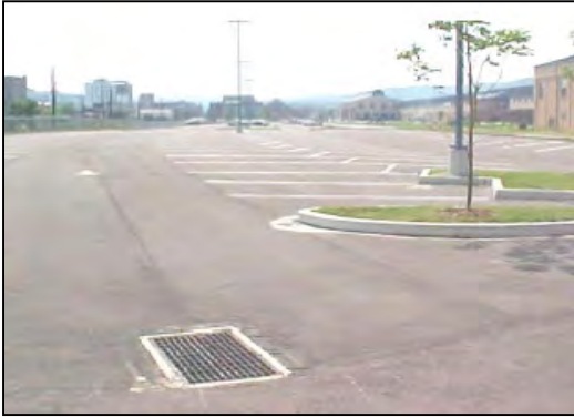
Grate Inlet in Parking Lot
