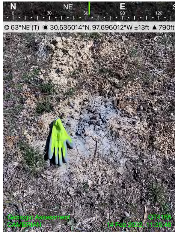
Photo 2. Filled geotechnical borehole on the site.
