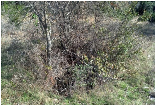
27. View of collapse feature (Geologic Assessment feature "S-1") located on northeastern portion of wooded area of property.
