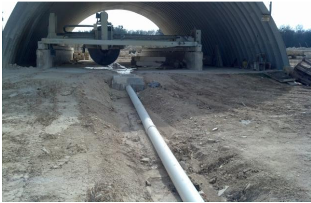
21. View PVC line located behind saw hut.
