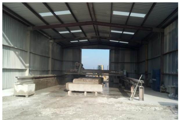
4. Interior view of fabrication building.
