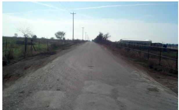
8. View looking south down CR305 in front of northern quarry entrance/exit.
