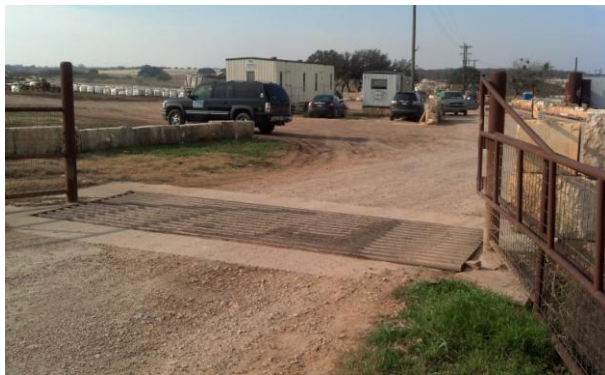
11. View of rumble grates at northern quarry entrance/exit.
