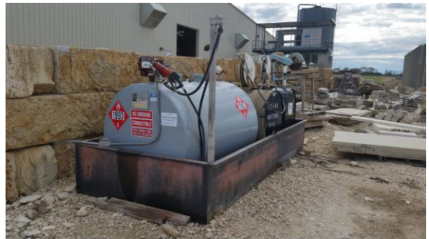
6. View of 500-gallon diesel fuel AST and two (2) 275-gallon motor oil ASTs located at northwest corner of fabrication building.
