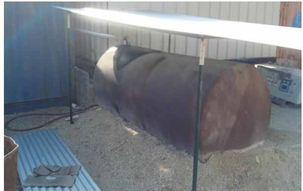
16. View of 600-gallon used oil AST located outside of maintenance area shed in Photo #15.
