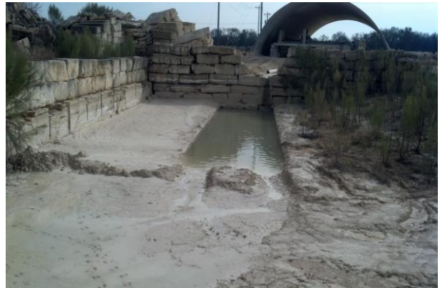
22. View of settling pond (to be decommissioned) located behind saw hut.
