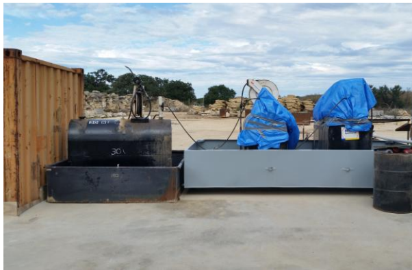
15. View of motor oil ASTs located in quarry maintenance area.
