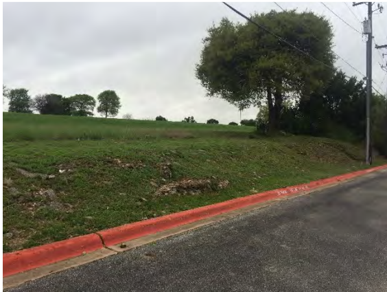
Entire length of zone of fractures looking to the north with I-35 in the background
