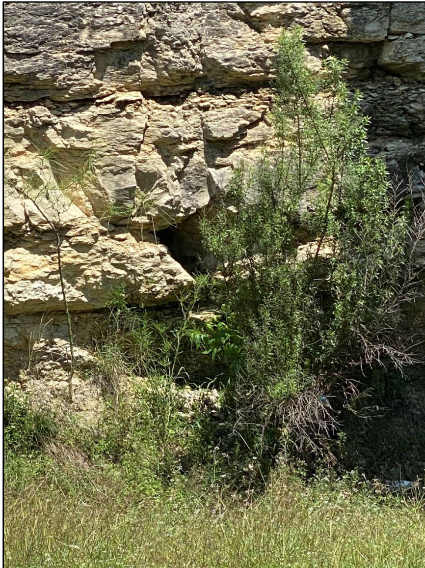
Feature Photo MPS-20 Solution Enlarged Fracture (Photo 2 of 2). The solution cavity associated with this fracture (center of image) is about 5 feet above the flow line at the base of the cliff.
