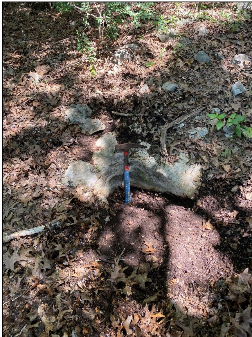
Feature Photo MPS-32 Solution Cavity.
