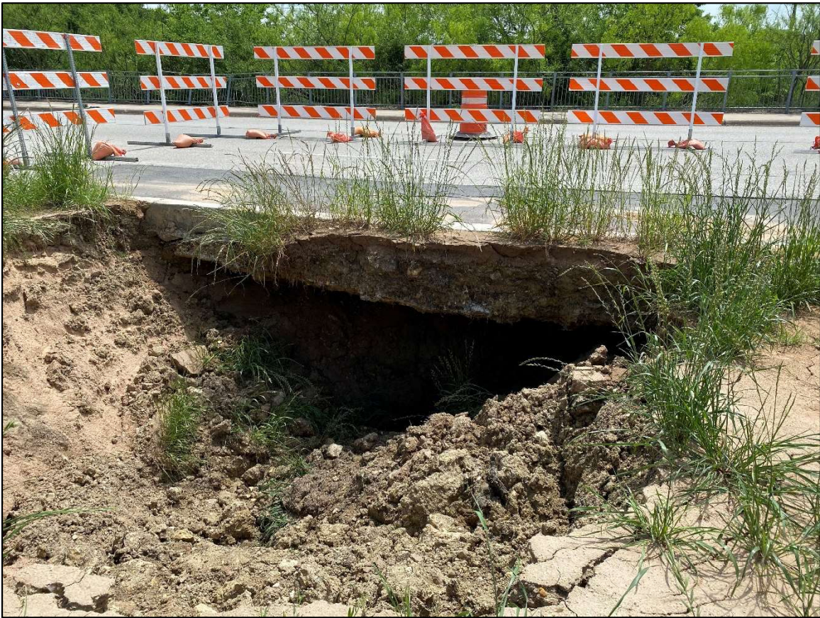
Feature Photo MPS-33 Non-karst Closed Depression (Photo 2 of 3). The depression was not excavated or probed due to the risk of further collapse. Photo taken on April 8, 2020.
