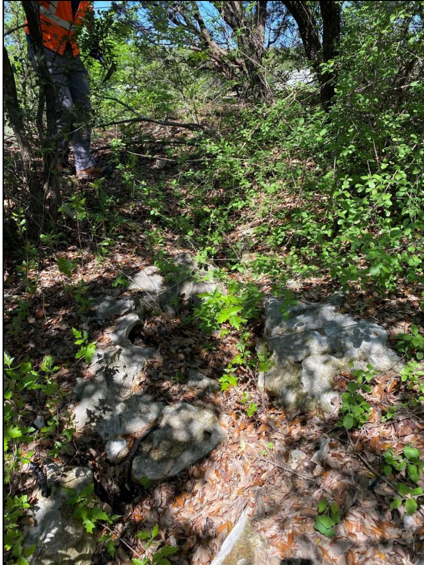
Feature Photo MPS-19 Solution Enlarged Fracture (Photo 1 of 2). The 27-foot long fracture is situated on top of a pinnacle. The fracture is partly covered with leaves. It runs between the two limestone slabs in the lower part of the image, to the right of the person standing for scale.
